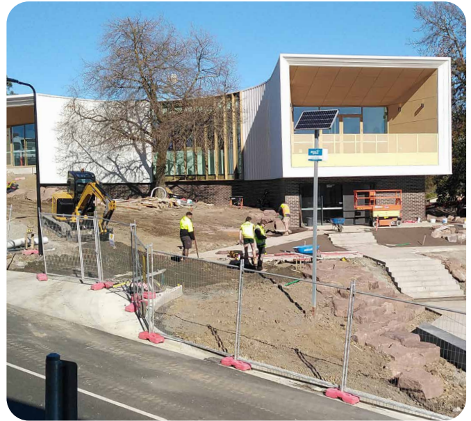
Above: Construction nearing completion at the Korumburra Community Hub.
